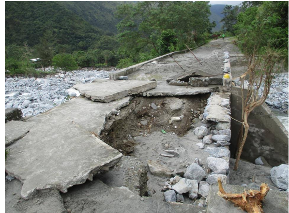
Damaged road in Dalupirip, Itogon. CORDIS-RDS Photo
